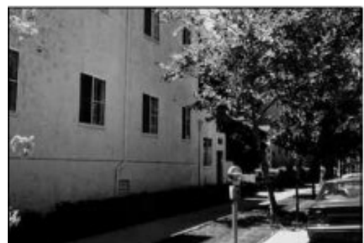
Above: UNDESIRABLE These apartment buildings have ground level parking and a tall blank wall along the street. The design is out of scale with the adjacent buildings. The architecture is spare and unattractive.
