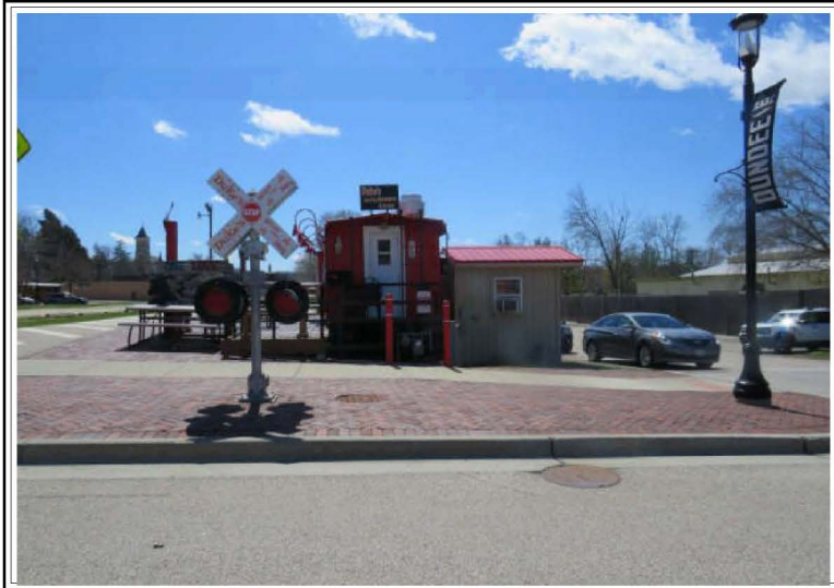
Front looking south
