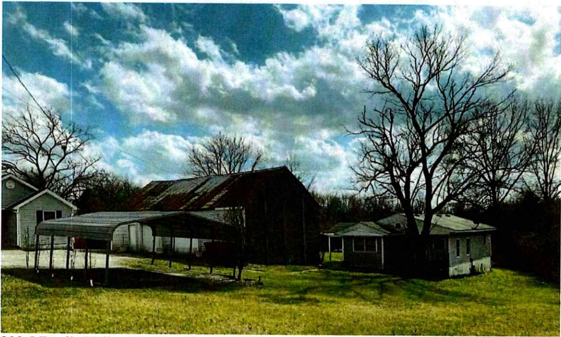
209.5 Devils Hollow Road and out-buildings
