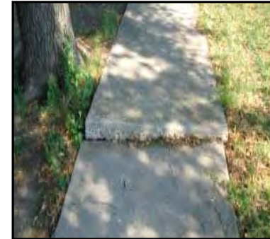
Surface roots have raised the sidewalk.
