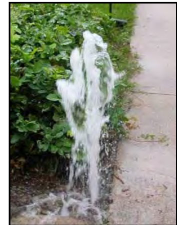
Broken sprinkler heads can waste water at the rate of 10 gallons per minute.
