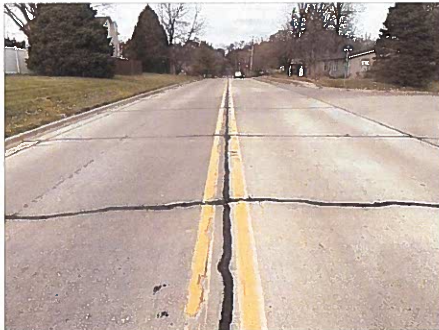
Location 2: Riggin Road north of Eagles Way
