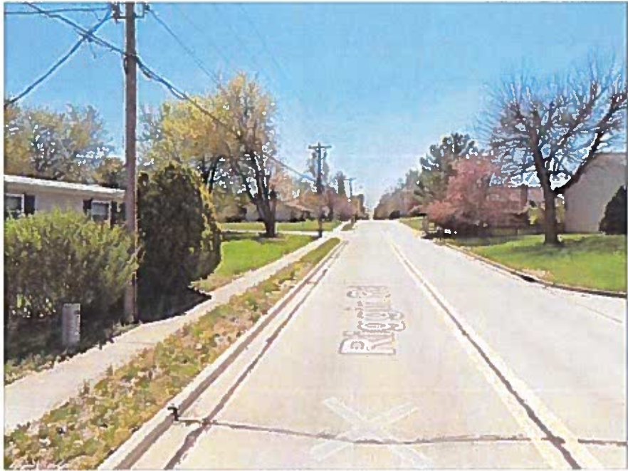
Photo 3: North Nottingham Rd looking south along Riggin Rd.
