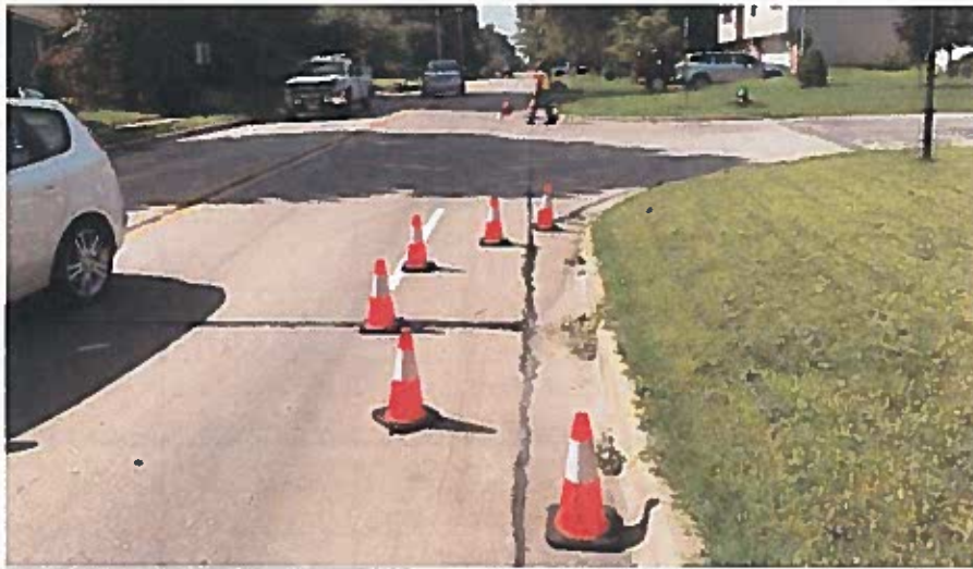
Figure 4 – Cones Used to Simulate a Curb Bump-out along Riggin Road.
