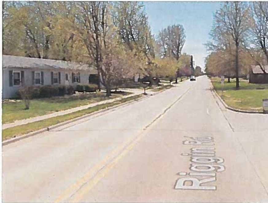
Photo 1: South Nottingham Rd looking south along Riggin Rd.
