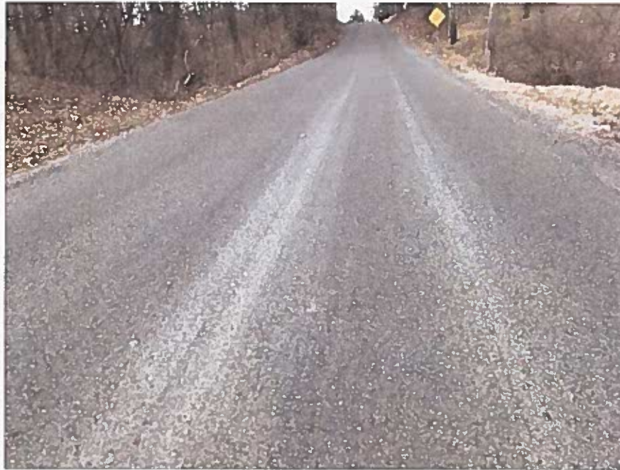
Location 3: Riggin Road north of existing bridge.
