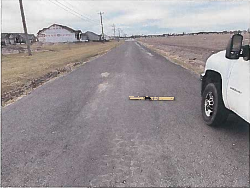
Location 3: Bouse Road west of Whitworth Drive
