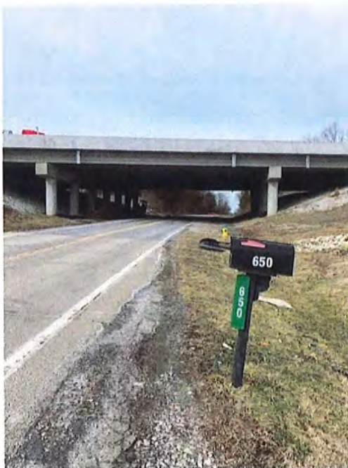
Looking North on KY-1665
