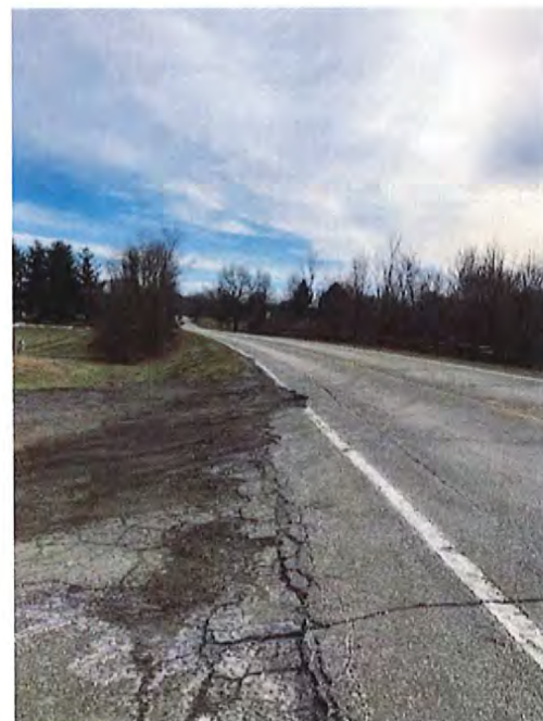
Looking South on KY-1665
