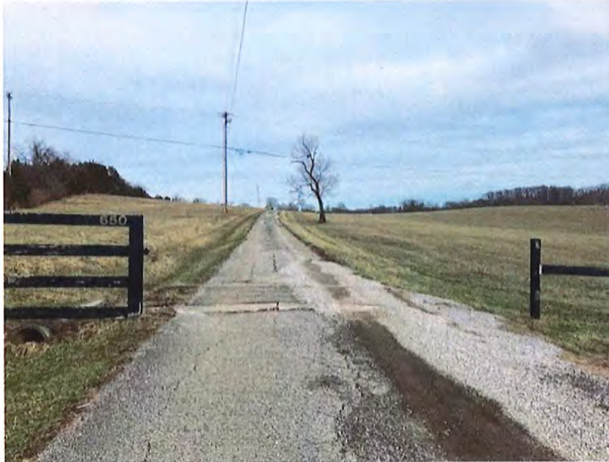
Entrance to property looking East
