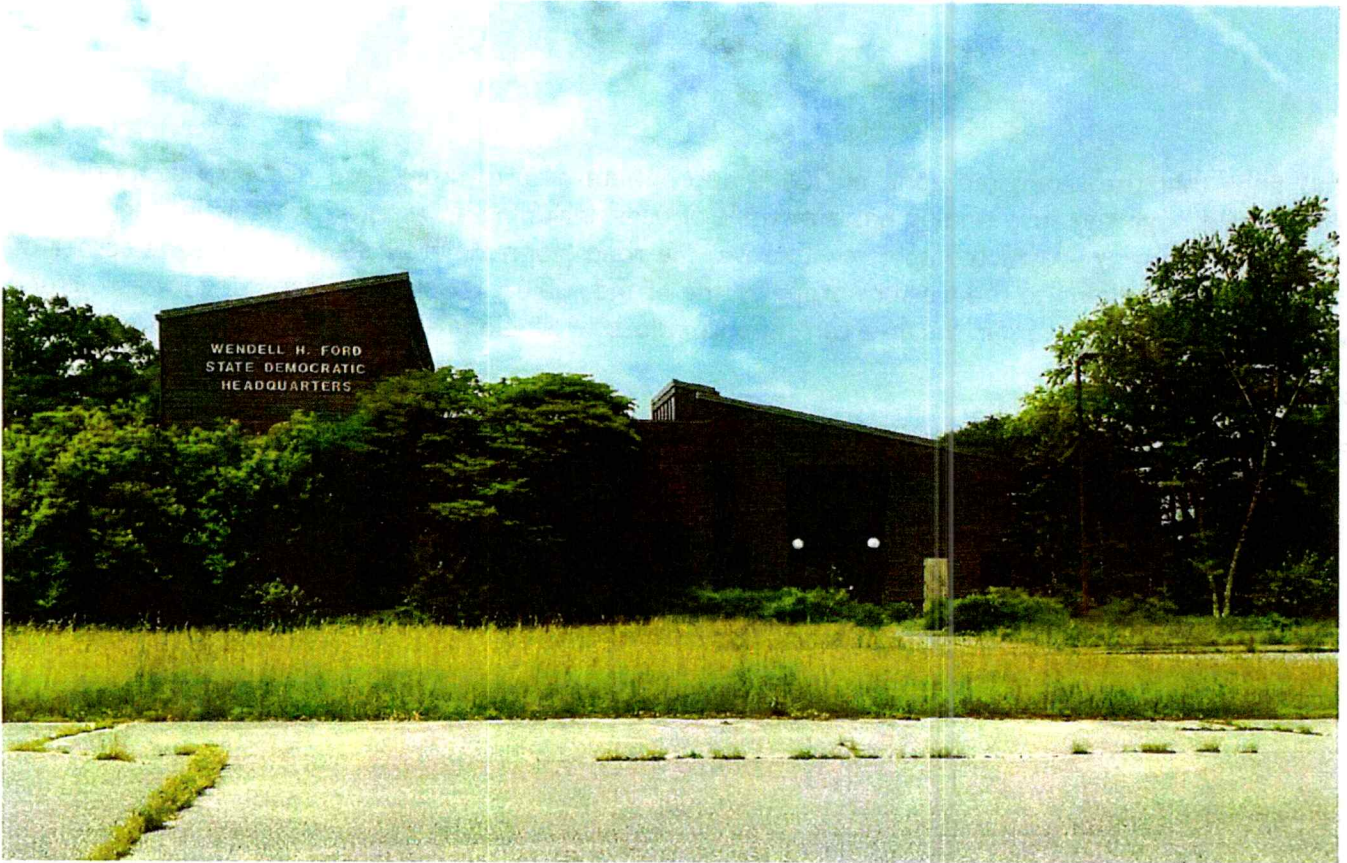
Existing structure on subject property
