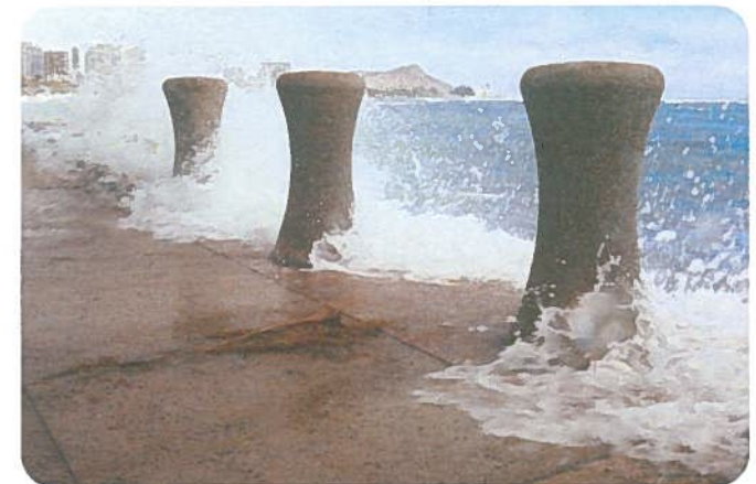
High wave overtopping at Kewalo Basin.
