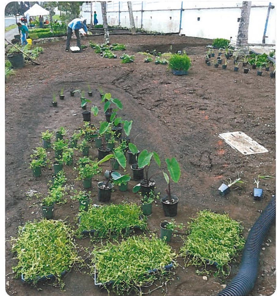
Example of a rain garden under construction at Windward Community College.
