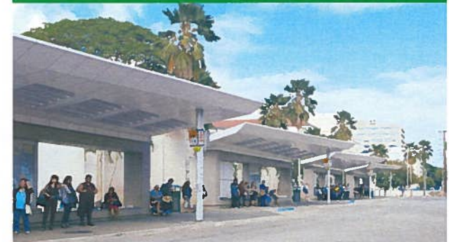
Bus-Only Lane on King Street (top); The Alapa'i Transit Center (bottom)
