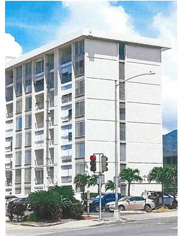
A multi-story midrise residential building.
