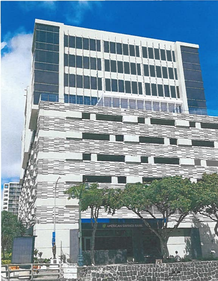
Parking structure screened by a decorative façade.
