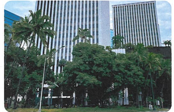
Downtown Honolulu commercial office buildings.
