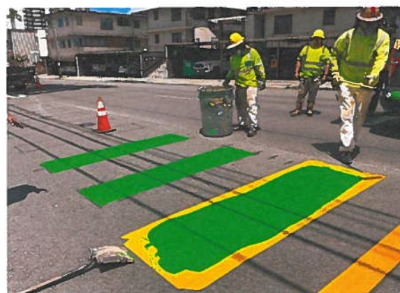
Construction of the Pensacola Bike Lanes (source: DTS)
