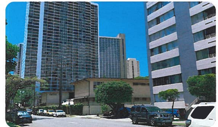
Small-scale projects have different needs than large-scale developments.
