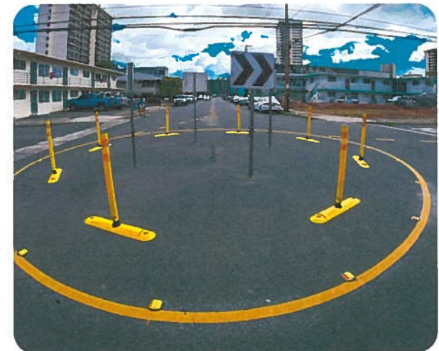
A mini traffic circle calms a McCully intersection (Source: DTS)
