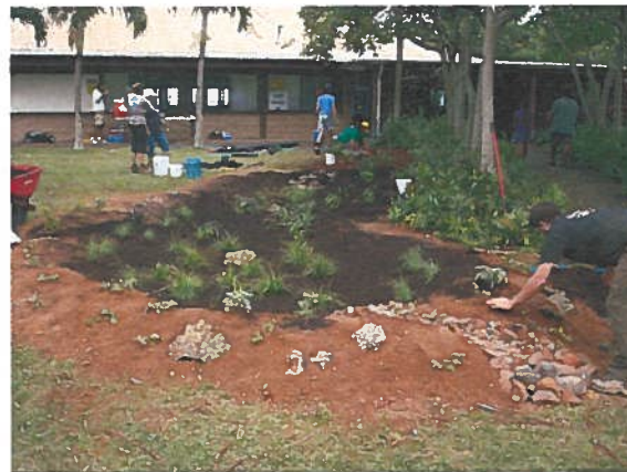
Green infrastructure to manage on-site flooding.
