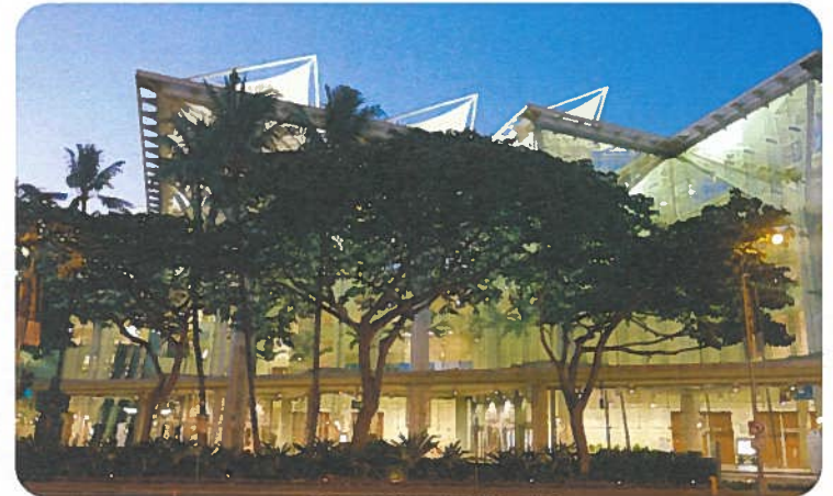
The Hawai'i Convention Center was designed with roof "sails" to maximize natural ventilation from the tradewinds, and an indoor-outdoor aesthetic.
