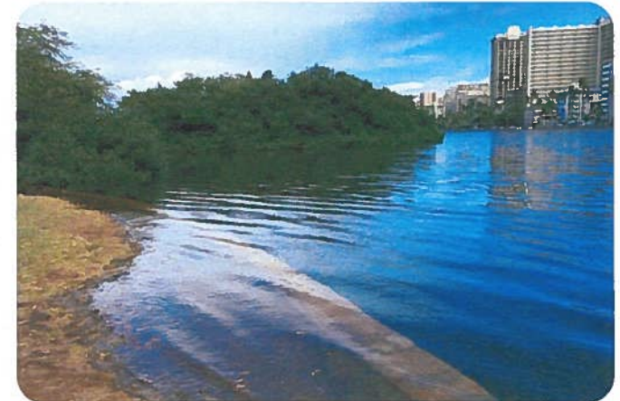
Ala Wai Canal overflow.
