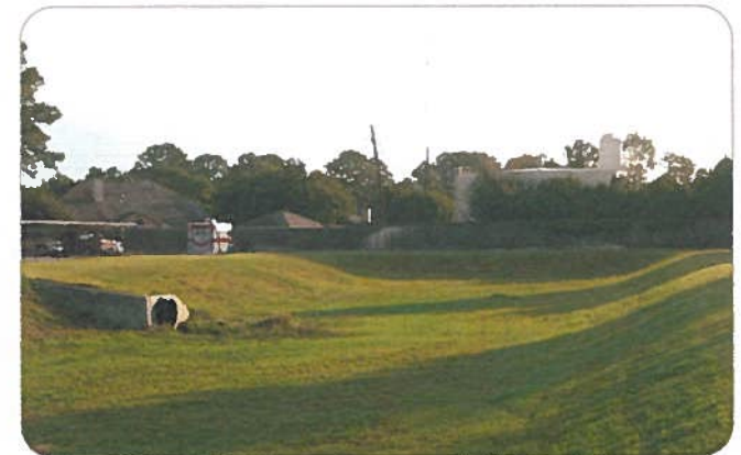
Example of a dry detention pond
