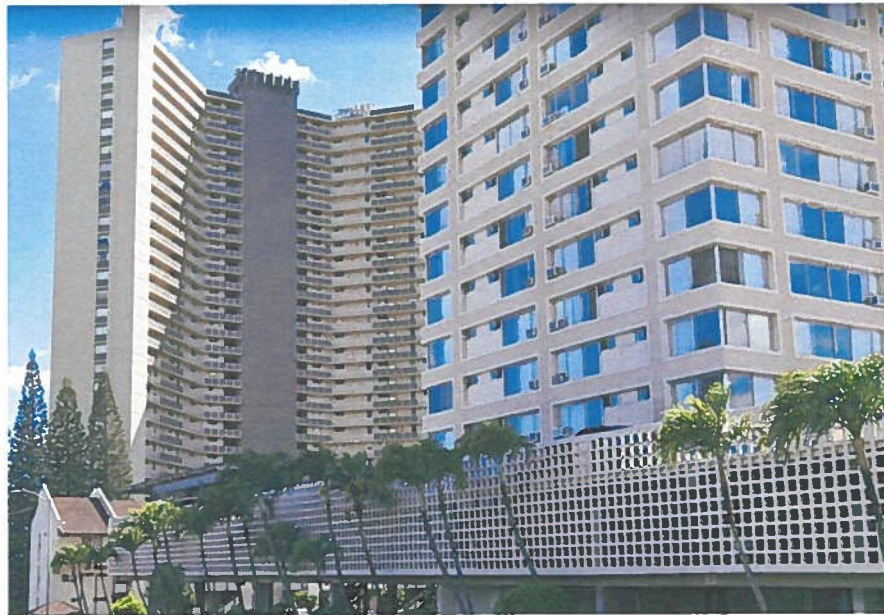
High density residential buildings around Pearlridge station area.
