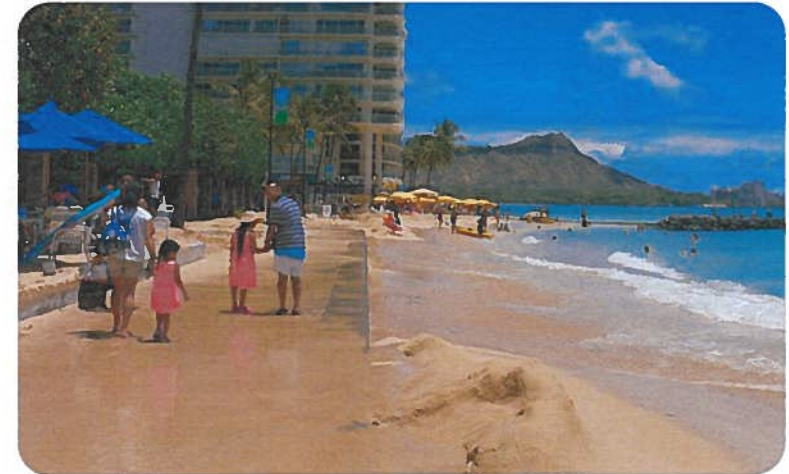
Engineered beaches in the PUC require maintenance against erosion.
