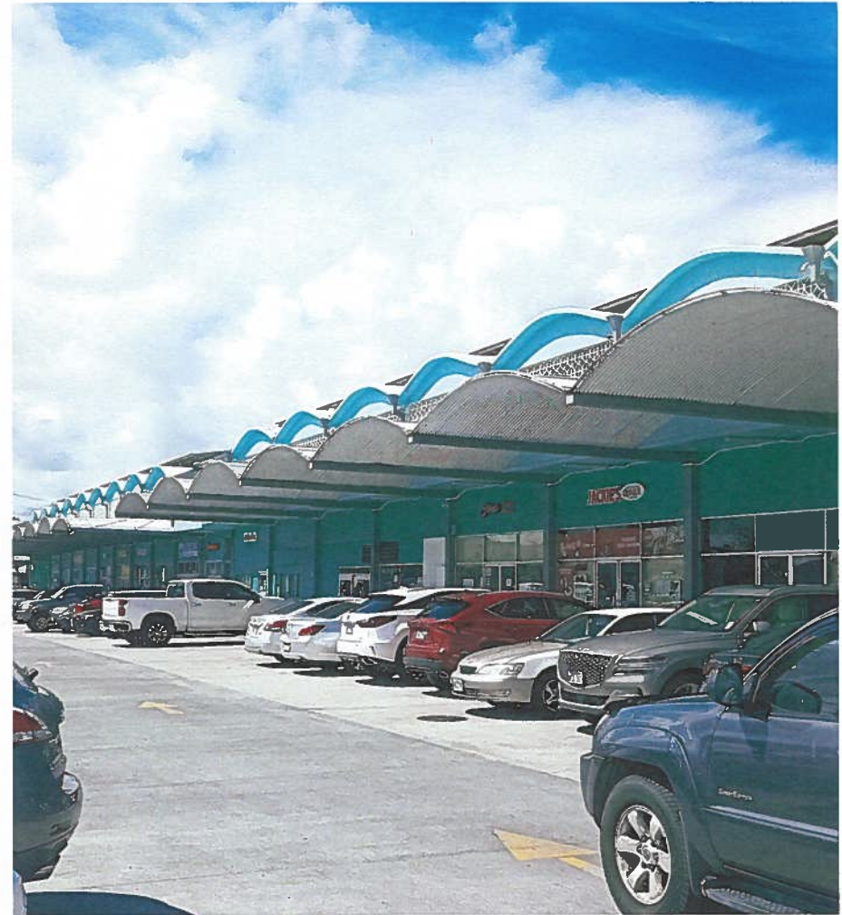
Community-serving retail stores at the historic Waimalu Shopping Center.
