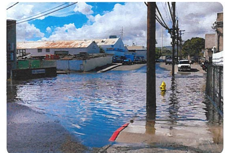
"Blue sky" tidal flooding in Kalihi Kai. (Source: UH Sea Grant King Tides Project)
