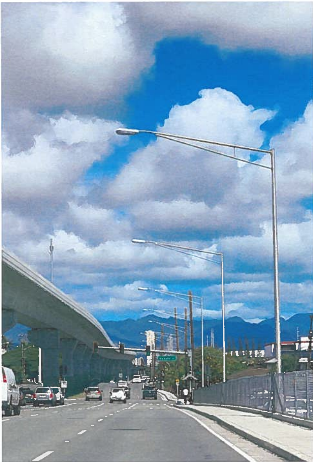
Elevated rail line along Kamehameha Highway.
