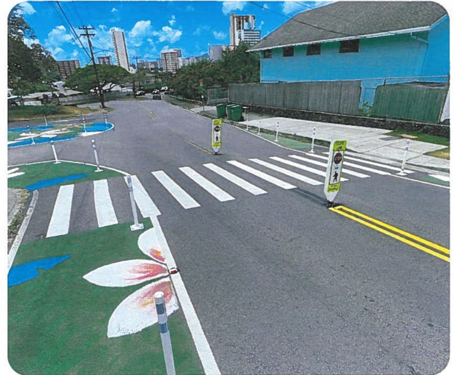
Pedestrian safety improvements near a school in the Punchbowl neighborhood (Source: DTS).
