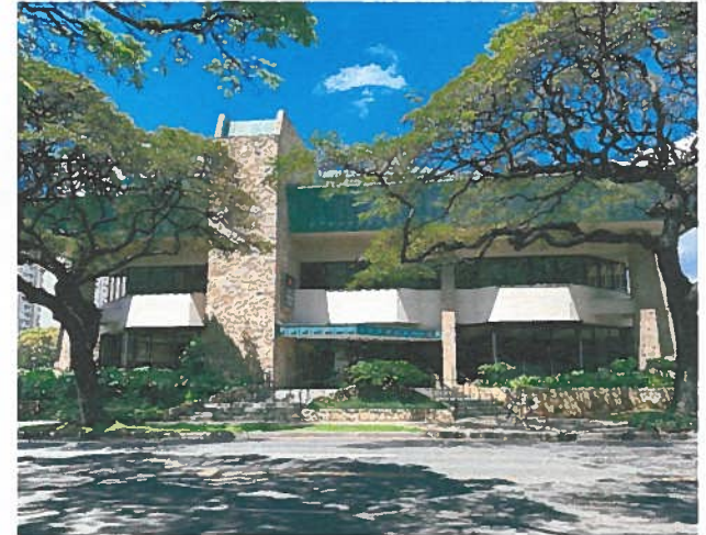
A Building well-connected to the public right of way.
