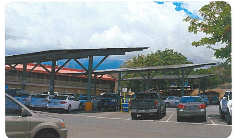
Solar panels over public parking
