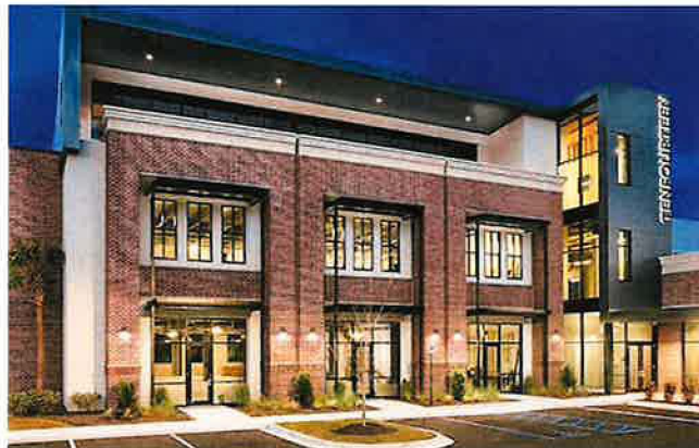
Use masonry as a primary building material and locate architectural elements (such as windows, doors, and roof lines) to express a rhythm of design.
